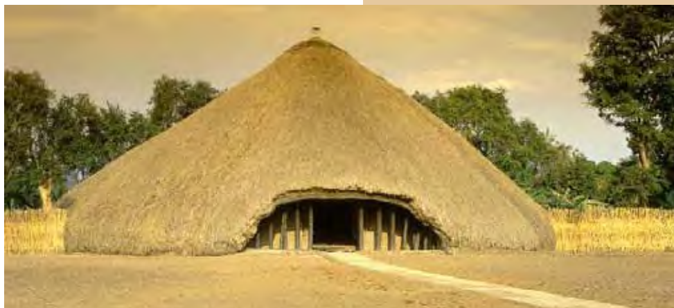
The original structure of Muzibu-Azaala-Mpanga building at Kasubi before fire outbreak
